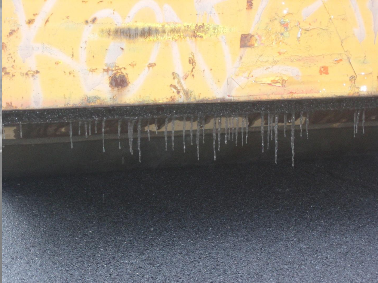
Icicles hanging from the back of the Hyster steel wheel compactor
